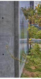
Panels mounted to new sub-frame attached to existing concrete wall
