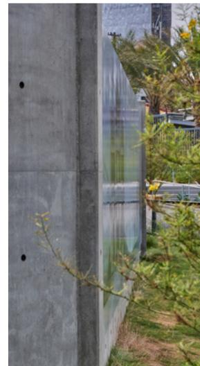
Panels mounted to new sub-frame attached to existing concrete wall
